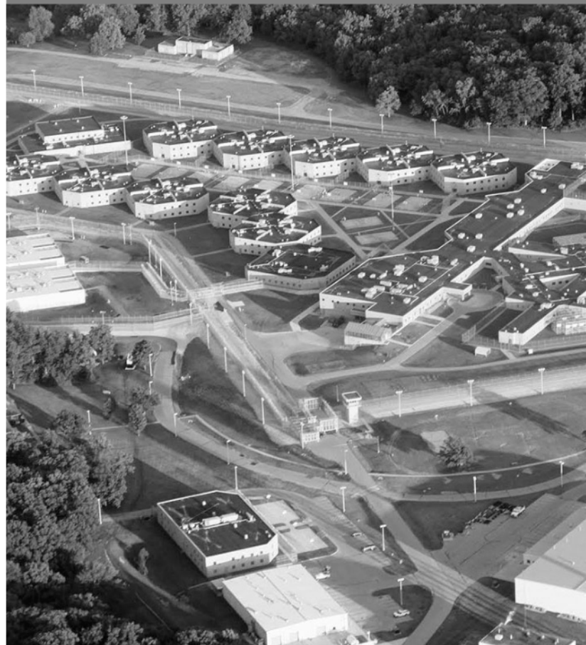
New Castle Correctional Facility PREA Recertified in 2019
