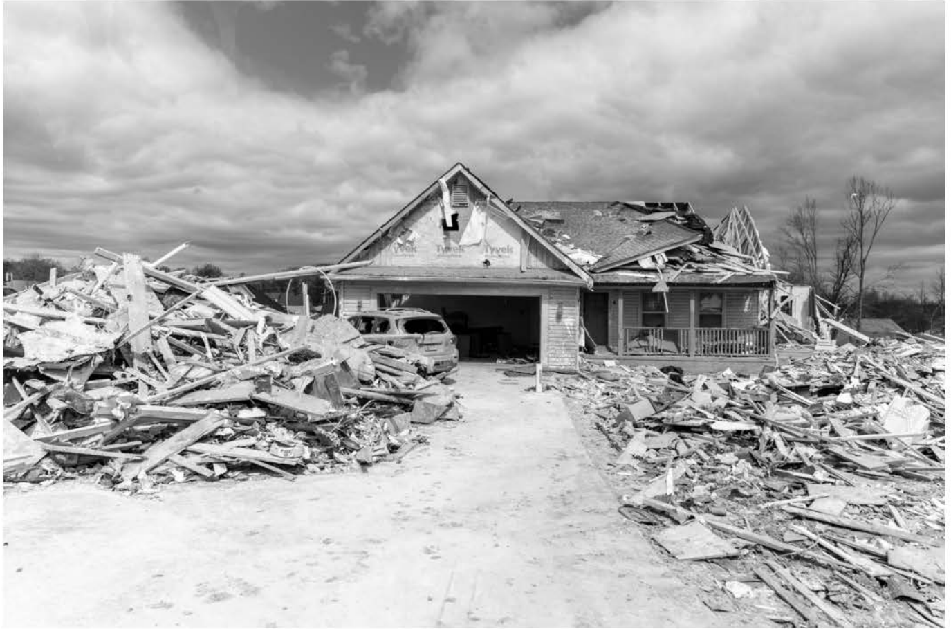
Damage caused by Tuesday's devastating tornado is seen during President Donald J. Trump's tour of a neighborhood Friday, March 6, 2020, in Cookeville, Tenn.. (Official White House Photo by Shealah Craighead)
